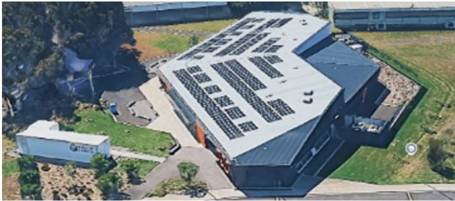
Wyndham Tech School solar roof.
