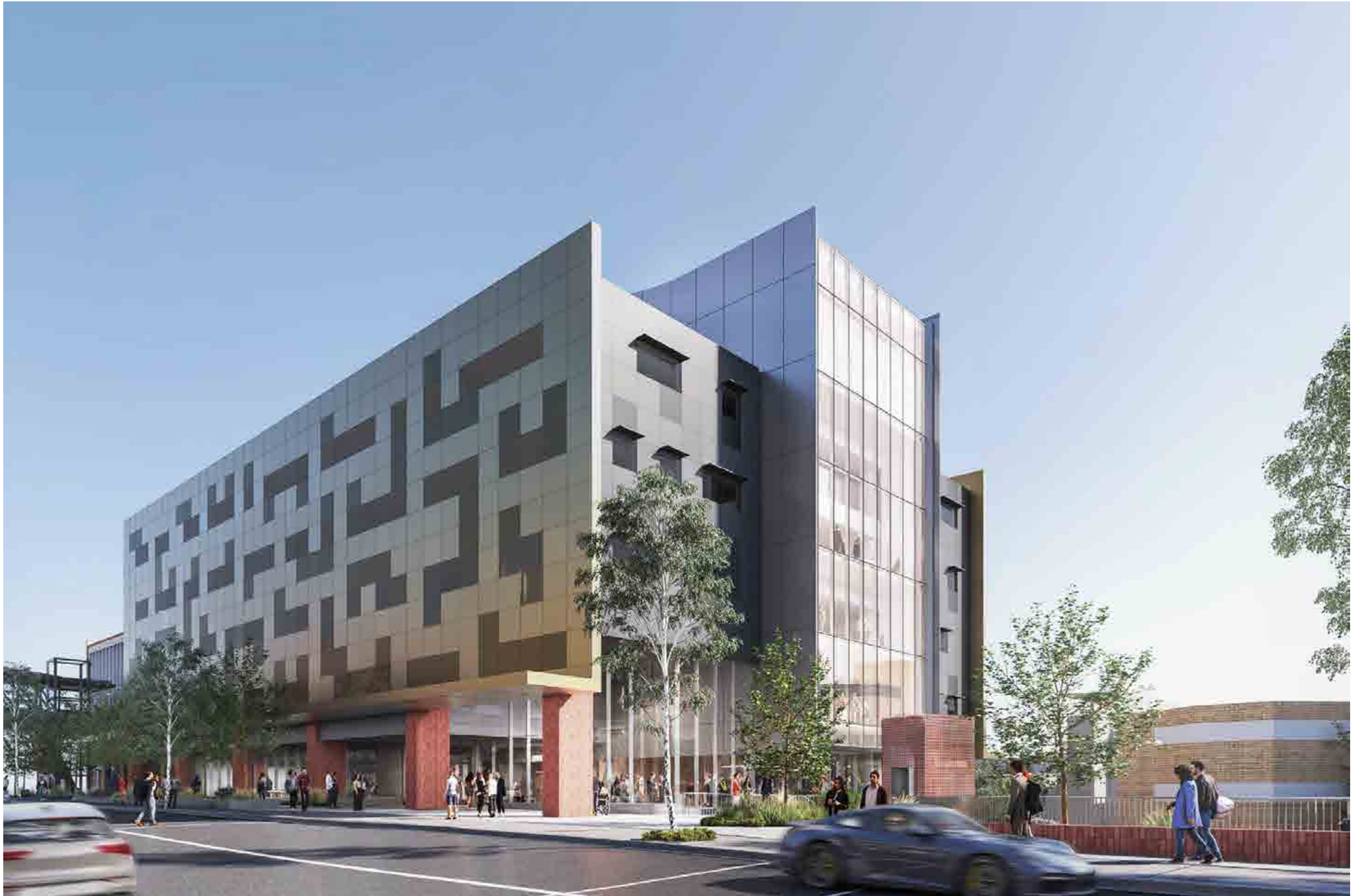
The articulation of the central spine and body clad with the L-shape plates breaks up the end volume to CHTF while the linear L-shape plates address the grander scale of the Ballarat Road frontage
