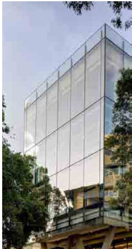
Specified glass has a low reflectivity and low body tint
