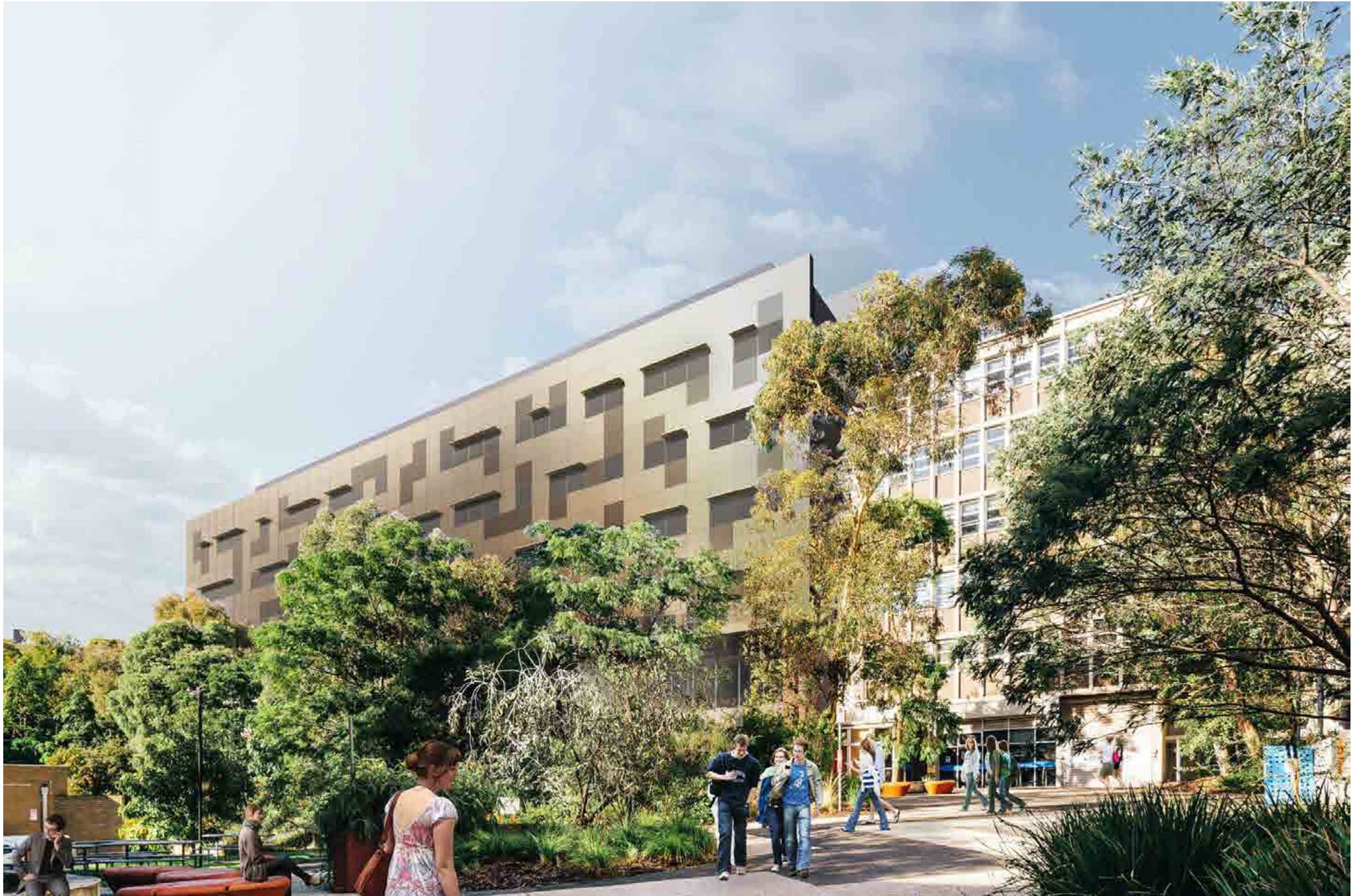
CHTF building forms a calm backdrop to the Footscray Campus Forest and creates outdoor areas sheltered from wind by the canopy of the L-shaped plate
