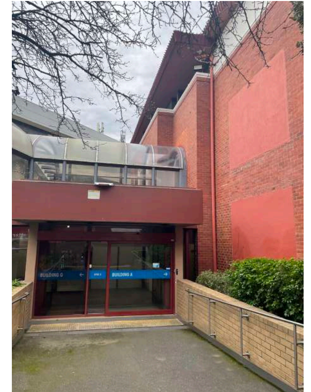
Link from south/Ballarat Road
