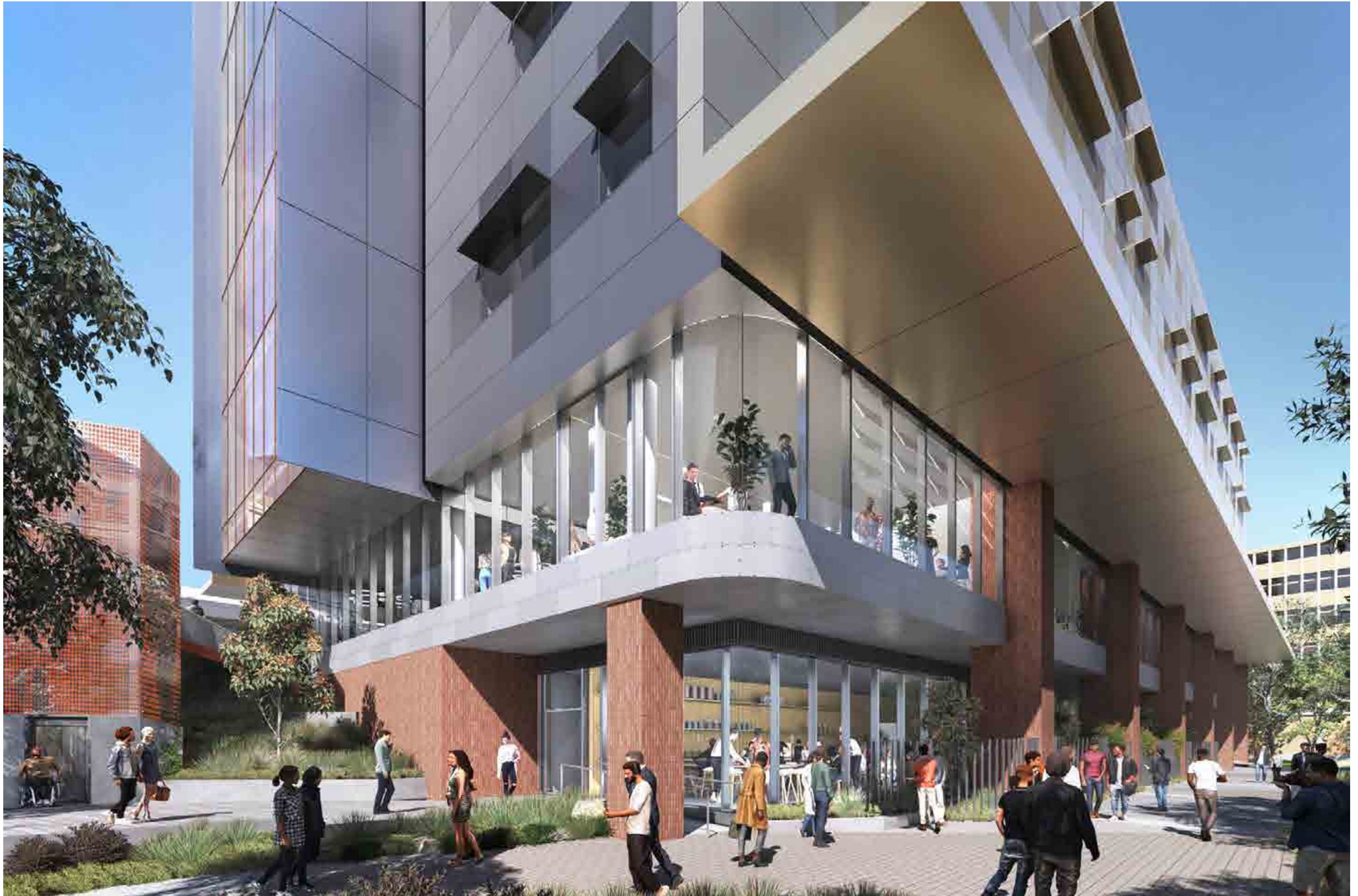
The large expressive brick piers ground CHTF into the campus and frame clear windows looking into education spaces and the cafe. These provide activation and passive surveillance to VU High Street and the Campus Gateway Park
