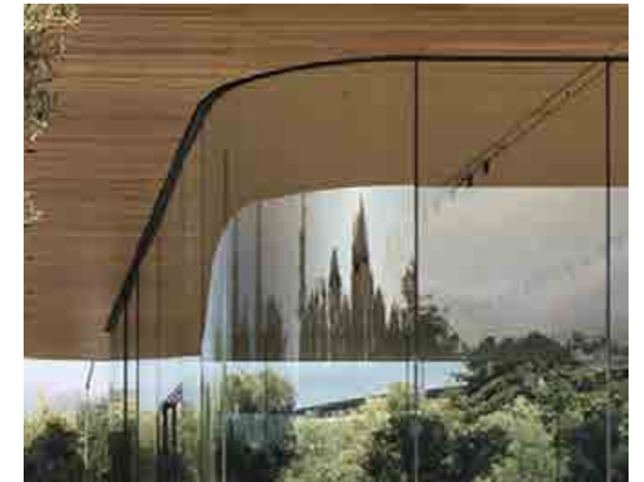
Curved glazed corner adding fluidity to the ground floor facade
