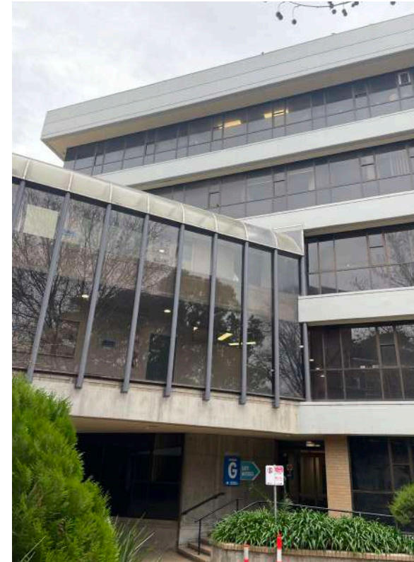
Link from east with existing entrance to Building G shown. Entrance to remain.
