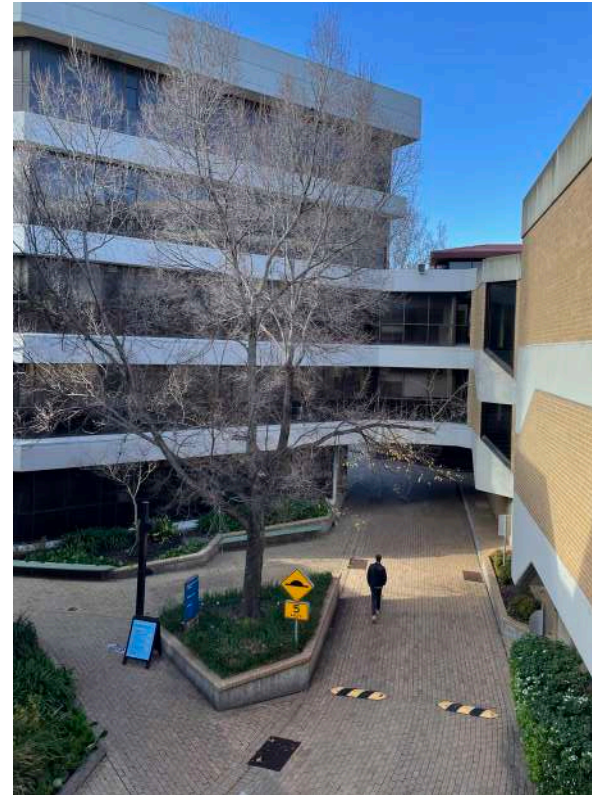
Existing conditions: Building G link over VU High Street from west
